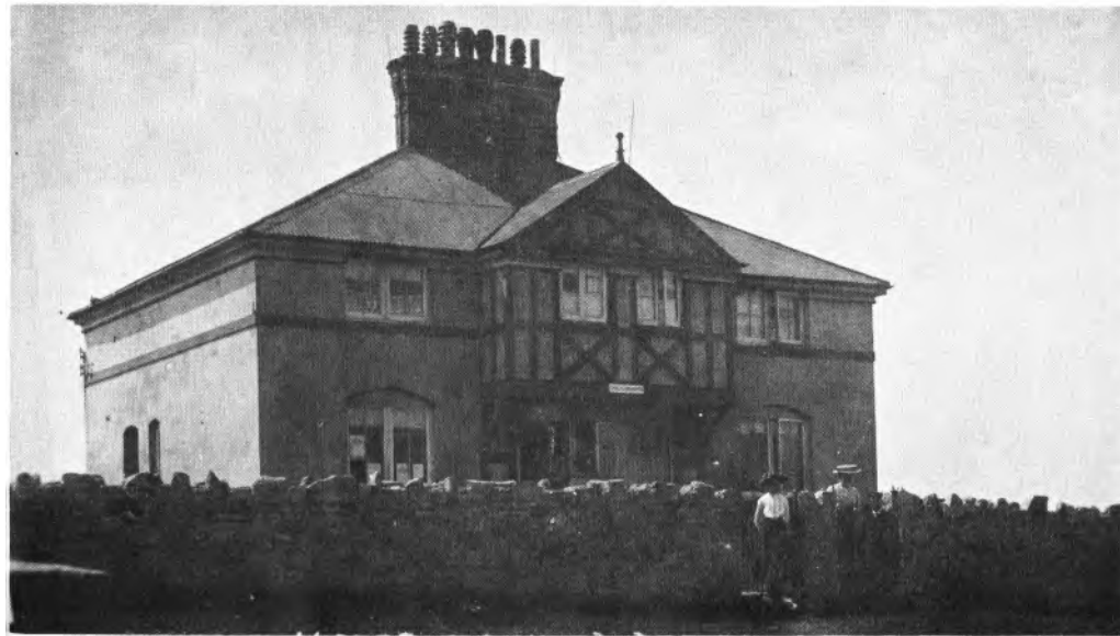
Left: Lloyd's Signal Station and British Sub-Post Office. The Post Office was located in the room on the left—the familiar red letter-box occupying a space in the bottom left-hand corner of the front window. The submarine cable from Hartland ended here, and it was from this office that the Rev. Hudson Grosett Heaven despatched his celebrated first message: "The Kingdom of Heaven rejoiceth".
