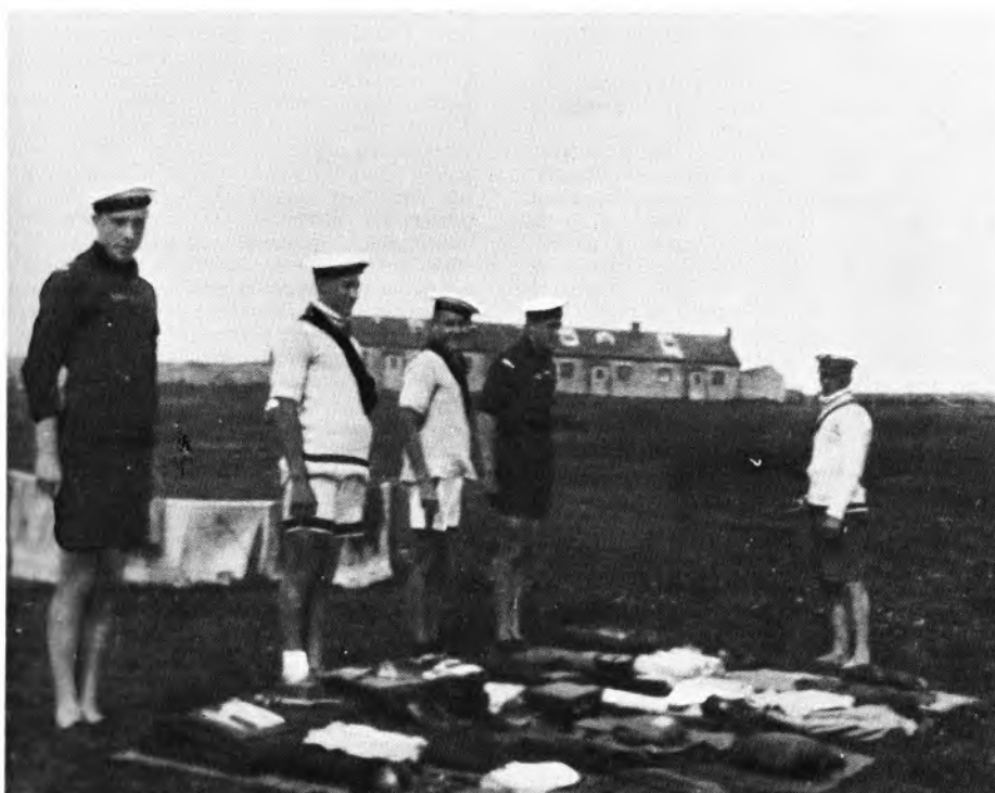
(Above) Kit inspection, 1928. Note the hipped roof of Barton Cottages in the background.
