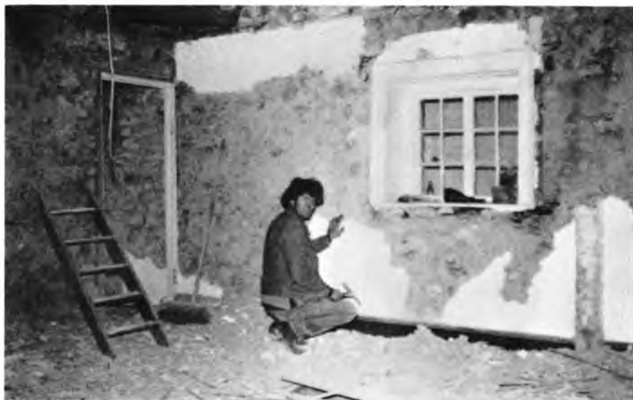
(Below) Work proceeds on gutting the middle section of the top floor in the old Hotel. Mr. Syd Allen works amongst the debris in what used to be room 22, and part of the corridor.
