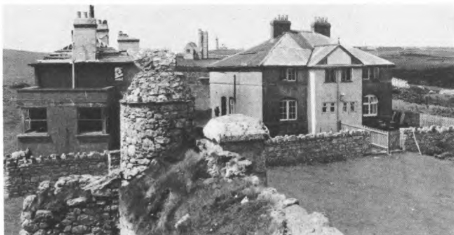
The Watch Room, Coastguard Cottages; and Signal Cottages, from the Castle ramparts in 1970. St. Helena's Church and the Old Light in the background. (Colin Taylor)
