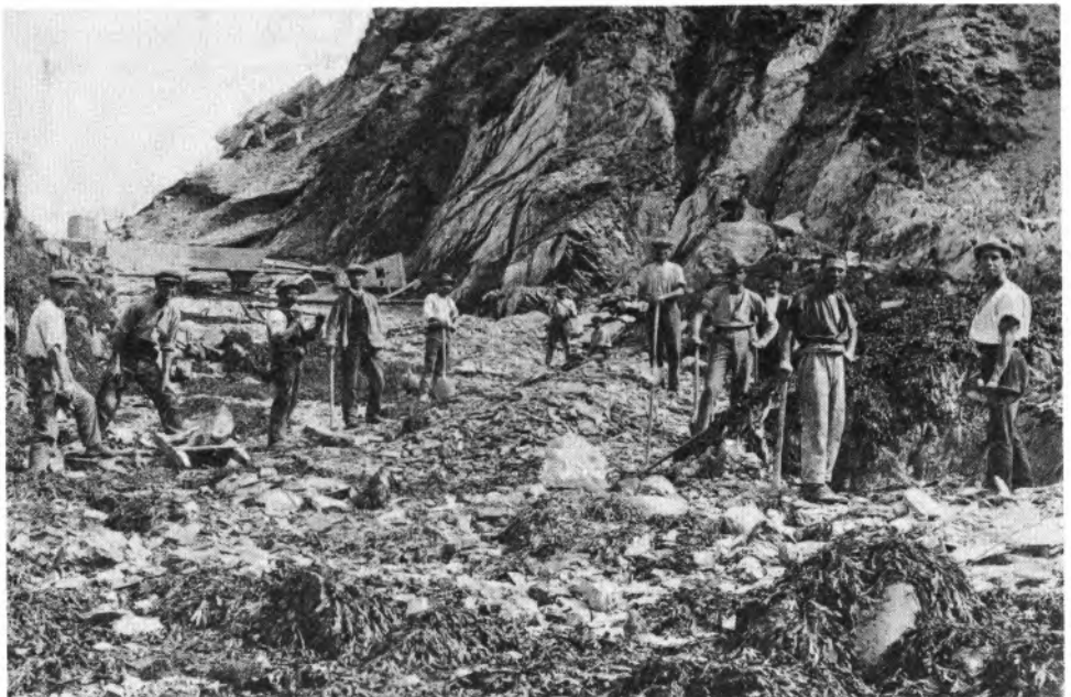
The Lundy Works. Ex-servicemen constructing the pier at the cove
